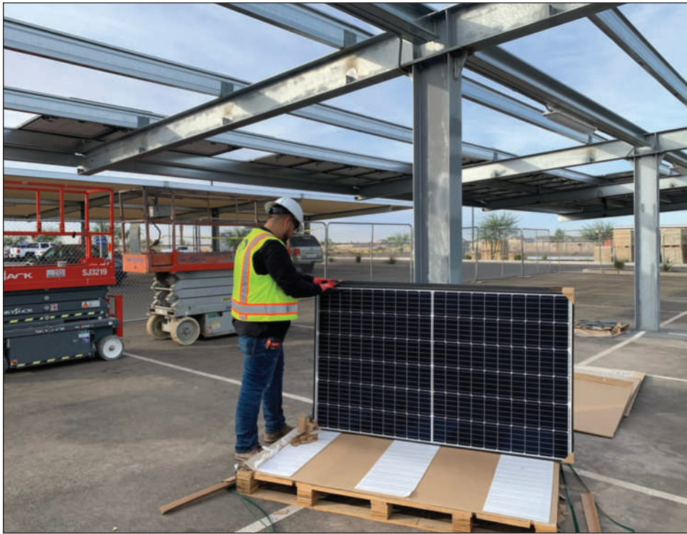
Brian Riveria works in the 351-kilovolt photovoltaic parking structure that Pilkington put up for San Luis Medical Mall.
